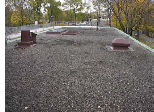
S45-003-R-CampbellPk View of roof
